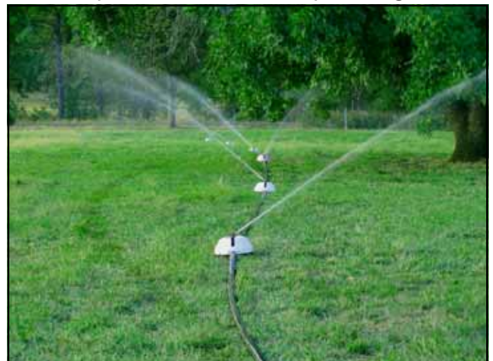
Irripod installed and operating:
