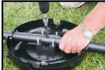
Drill 15mm or 9/16" hole and remove all drilling swarf.
