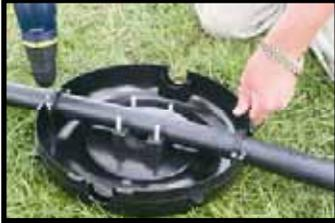
Lay pipe over Skid base and Cross Tee Anchor (check orientation).
