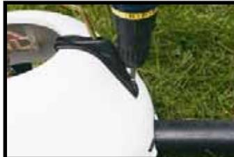
Screw the wire clip holders into the holes provided.
